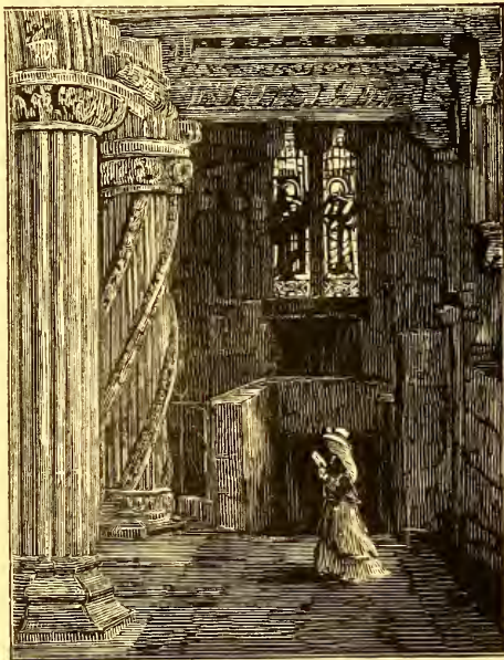
APPRENTICE PILLAR—ROSLIN CHAPEL.
